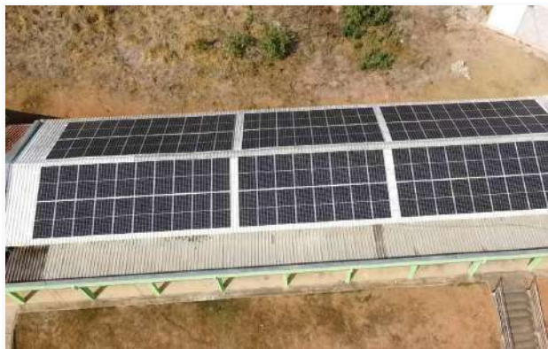
Figure 21: Machado Campus implementation of new photovoltaic modules.
