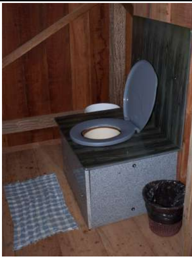
Figure 23: Inconfidentes Campus dry toilet at Agroecology Sector.
