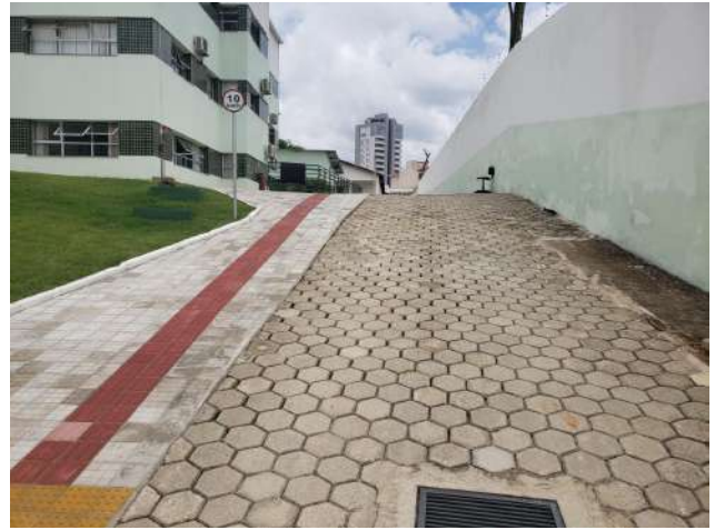
Figure 30: Rectory renovation of the drainage system.
