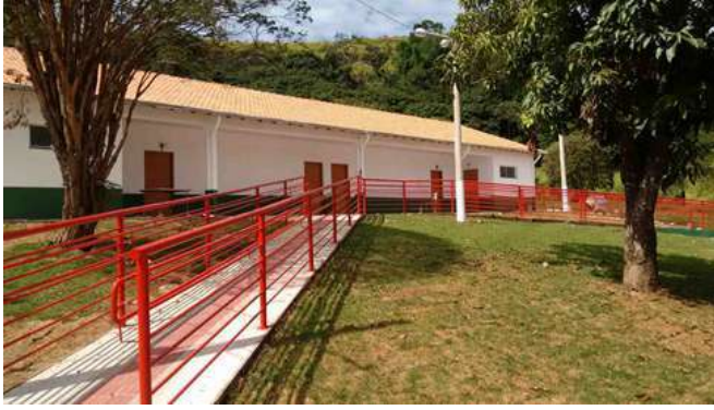
Figure 5: Carmo de Minas Campus tactile paving and handrails.
