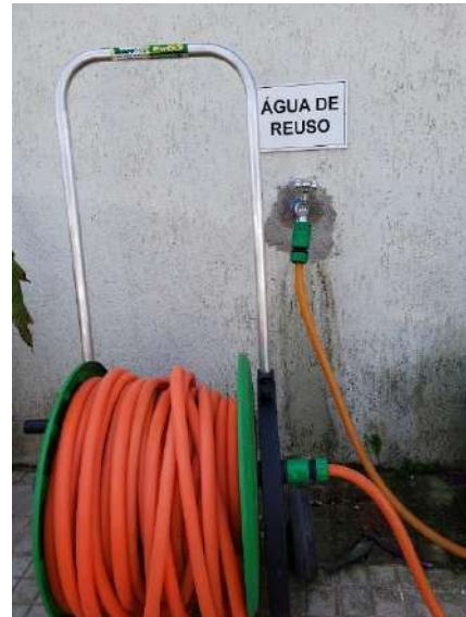
Figure 18: Rectory sign indicating reused water tap.
