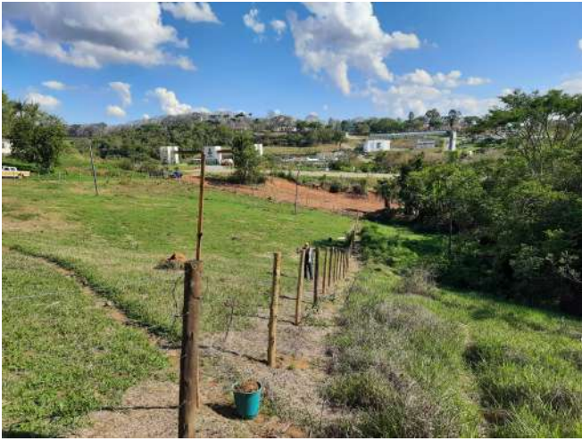
Figure 22: Machado Campus fencing and planting trees to recover water sources.
