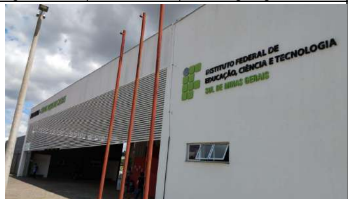
Figure 20: Campus Poços de Caldas building facade brise-soleil.
