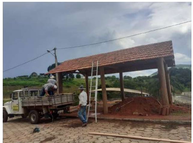
Figure 34: Inconfidentes Campus construction of living space using used materials.
