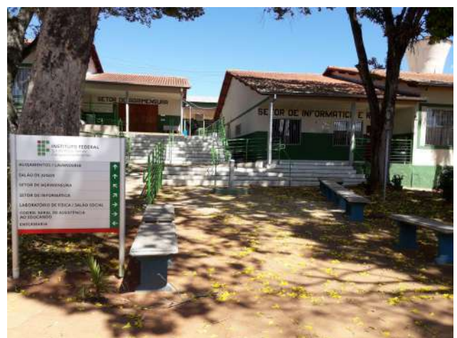
Figure 18: Inconfidentes Campus sector indication board, ramps and handrails.
