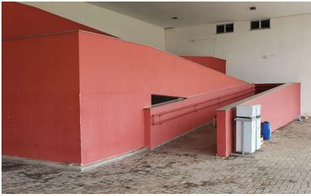
Figure 13: Poços de Caldas Campus ramp and handrails.
