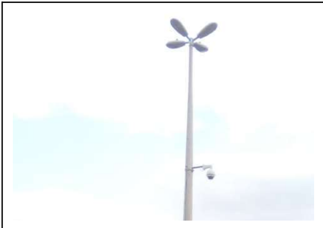
Figure 1: Machado Campus 360° monitoring camera.
