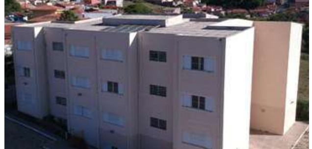
Figure 26: Inconfidentes Campus Visconde de Mauá student building solar heating system.
