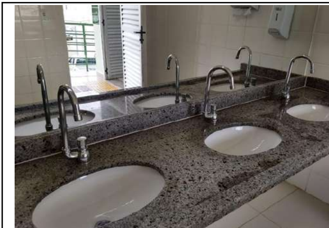
Figure 1: Rectory time delay water taps.
