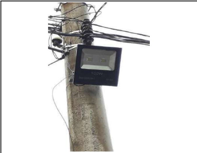
Figure 11: Campus Carmo de Minas high-efficiency luminaires with automatic lighting control – LED lamp post.
