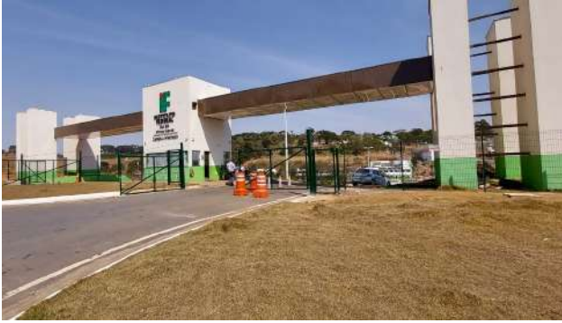
Figure 11: Machado Campus entrance closed with railings.
