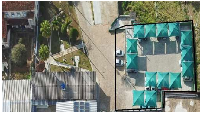
Figure 4: Carmo de Minas Campus parking lots.
