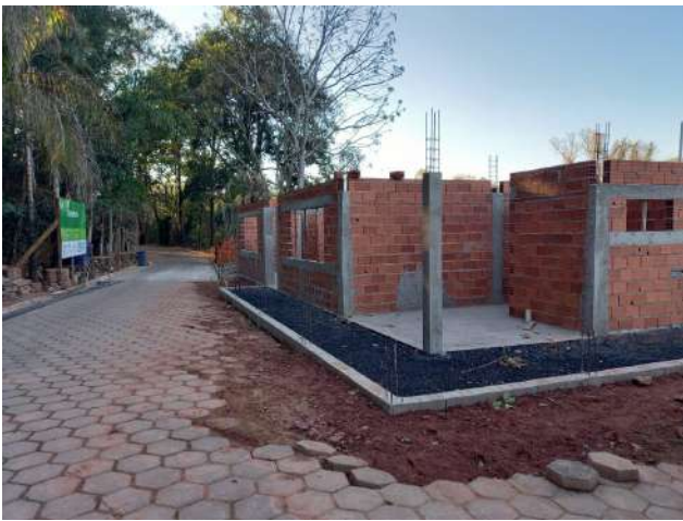
Figure 37: Inconfidentes Campus construction of the Hippotherapy Center building.
