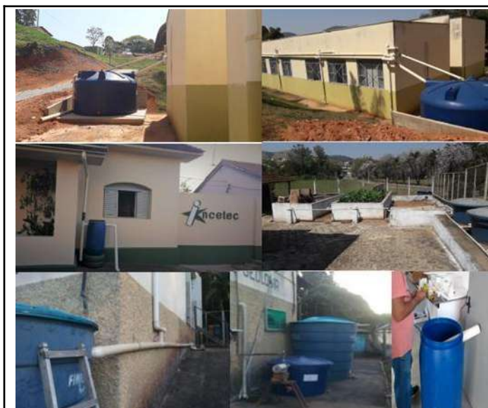
Figure 1: Campus Inconfidentes rain harvesting system.
