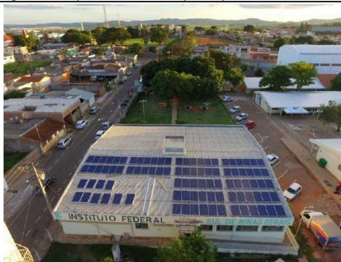
Figure 4: Campus Passos solar power plant.
