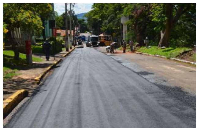
Figure 4: Machado Campus street paving refurbishment.
