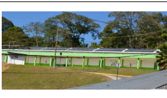
Figure 2: Campus Machado solar power plant.
