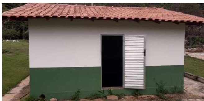
Figure 20: Carmo de Minas Campus water storage cisterns with a capacity of 80,000 liters.
