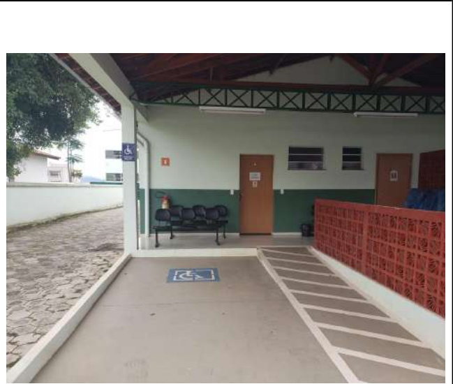
Figure 6: Rectory parking and ramp for people with special needs.
