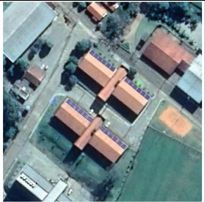
Figure 18. Muzambinho Campus Solar water heating system.
