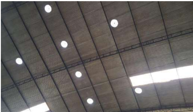
Figure 13: Campus Machado multi-sport gym roof natural lighting and exhausters.
