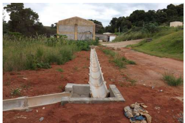
Figure 8: Machado Campus streets drainage.
