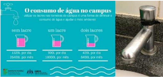
Figure 7: Campus Pouso Alegre tap with cable ties.
