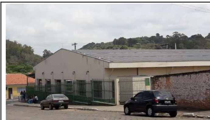
Figure 1: Campus Inconfidentes solar power plant.
