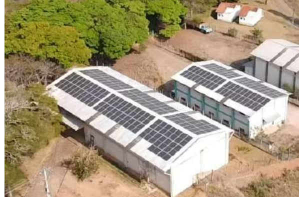
Figure 22: Machado Campus implementation of new photovoltaic modules.
