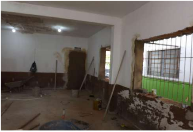
Figure 5: Machado Campus renovation of the Nursing Laboratory.
