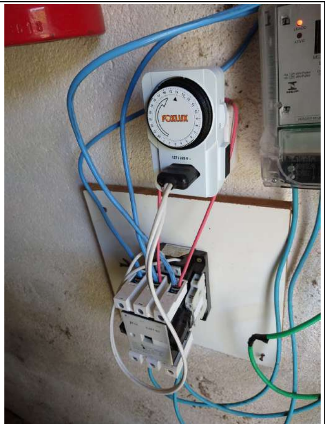
Figure 12: Machado Campus artesian well timer to turn off at peak hours and save energy.
