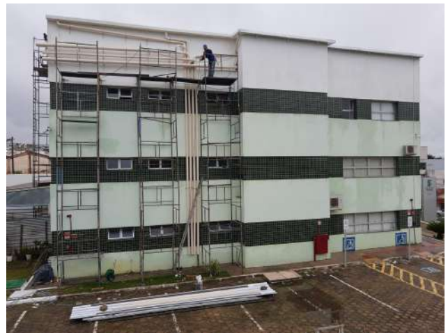
Figure 32: Rectory renovation of the rainwater collection system.
