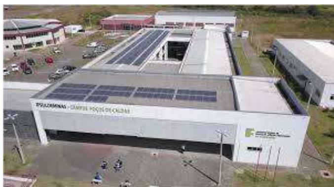
Figure 5: Campus Poços de Caldas solar power plant.
