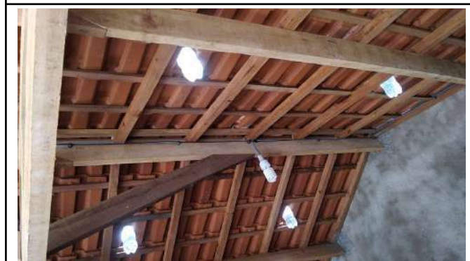
Figure 19: Inconfidentes Campus natural lighting with pet bottles filled with water.
