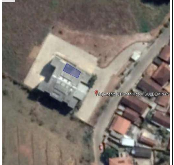
Figure 16. Inconfidentes Campus Solar water heating system.
