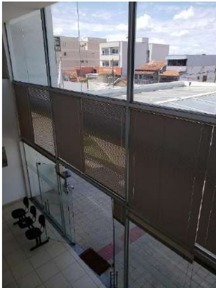
Figure 11: Rectory entrance natural lighting.
