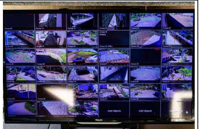
Figure 20. Inconfidentes Campus video surveillance system – Camera control.
