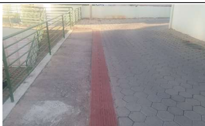
Figure 2: Rectory tactile paving.
