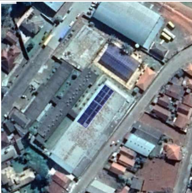
Figure 19. Muzambinho Campus CeCAES Solar water heating system.
