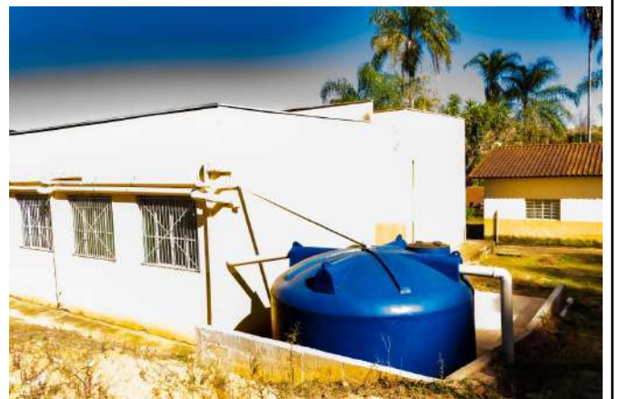
Figure 22: Inconfidentes Campus rainwater recovery system.
