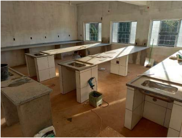
Figure 35: Inconfidentes Campus renovation of the Environmental Laboratory.
