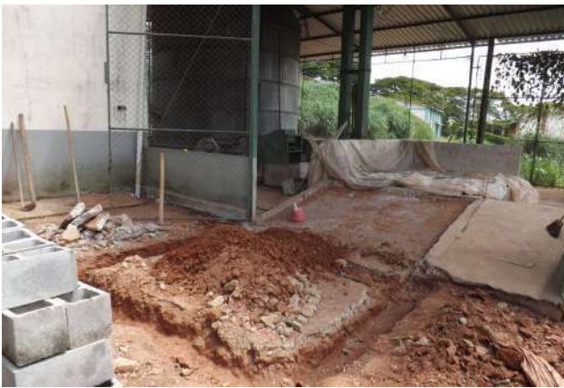
Figure 13: Machado Campus Feed Factory improvements.
