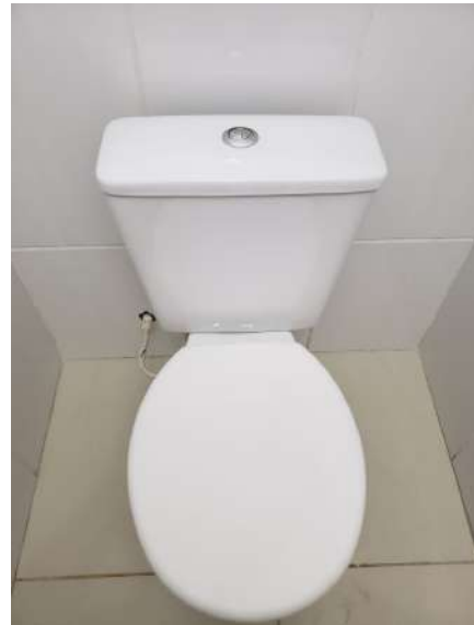
Figure 10: Rectory toilet flushing with double activation.
