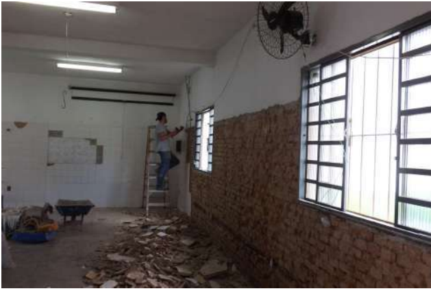
Figure 17: Machado Campus renovation of the Zoology Laboratory.
