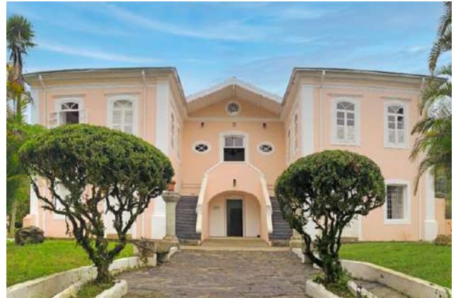
Figure 26: Carmo de Minas Campus Casarão old mansion renovated with its original architecture.
