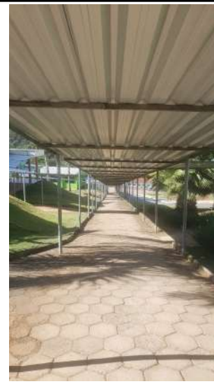
Figure 6: Machado Campus covered sidewalk.
