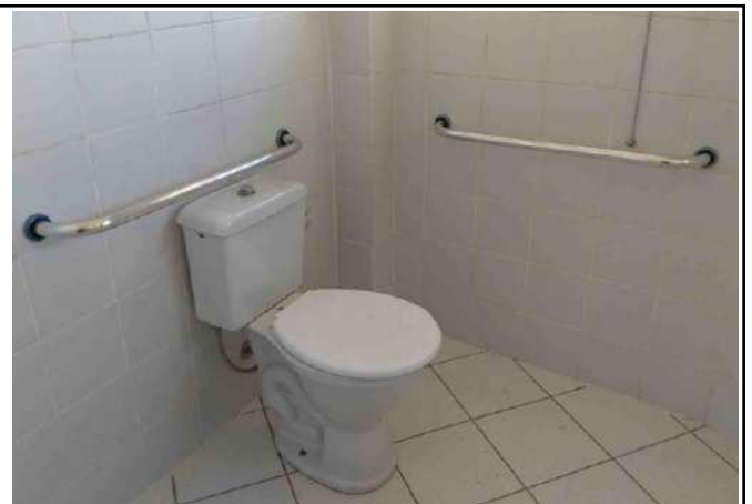
Figure 2: Rectory toilet water box flush.
