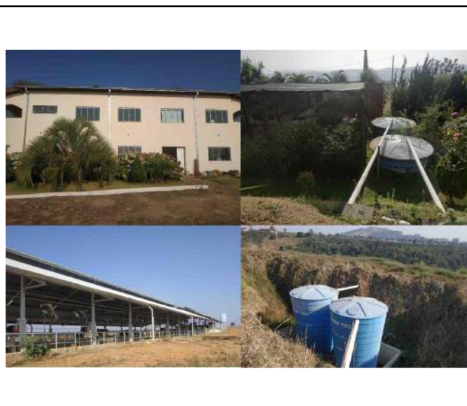
Figure 2: Campus Muzambinho rain harvesting system.
