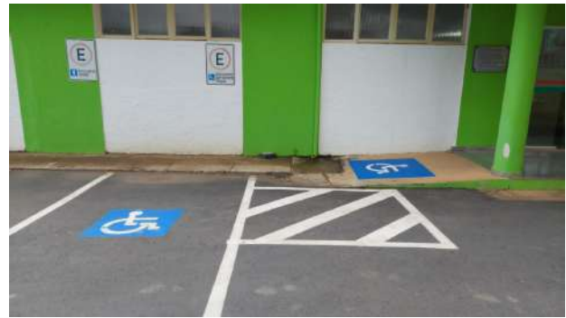
Figure 2: Machado Campus parking ramp for people with special needs.
