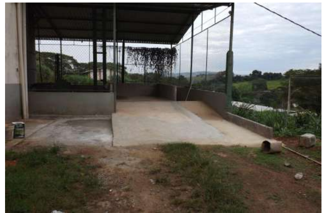
Figure 14: Machado Campus Feed Factory improvements.
