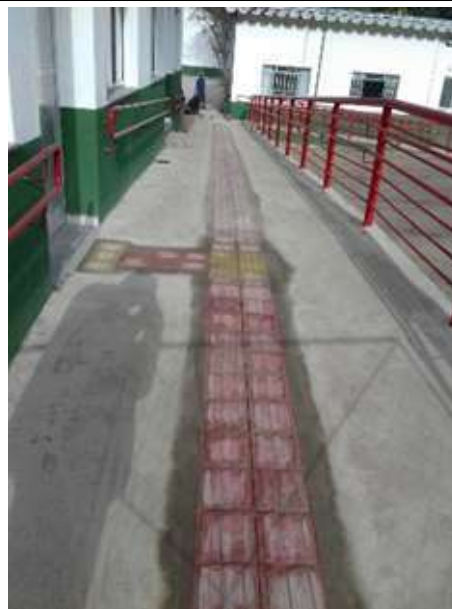
Figure 4: Carmo de Minas Campus tactile paving and handrails.
