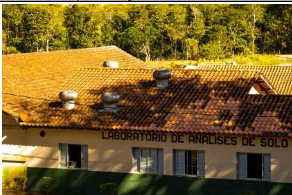
Figure 19: Campus Inconfidentes Soil Analysis Laboratory exhausters.
