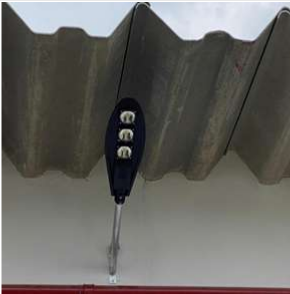
Figure 25: Carmo de Minas Campus lamp with photocell sensor.
