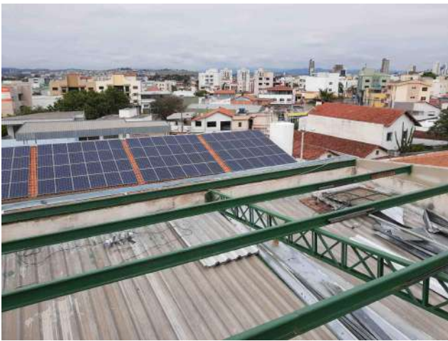
Figure 27: Rectory roof renovation.
