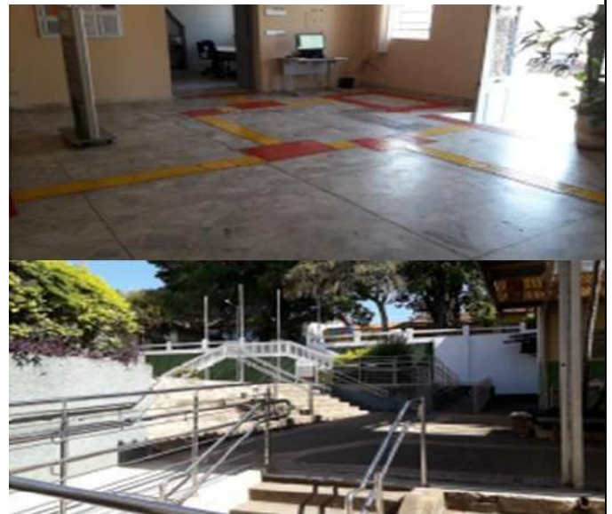
Figure 8: Inconfidentes Campus tactile paving, ramp and handrails.
